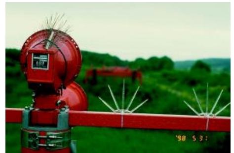
An anti-perch device can help reduce the attractiveness of an airfield to raptors.
